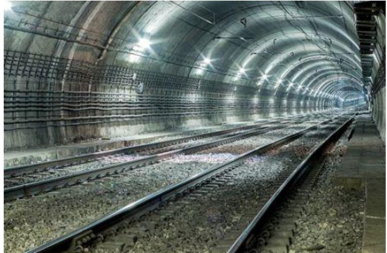
The existing rail tunnel beneath Hwy # 401 in the Toronto area (Source Infrastructure Ontario)
